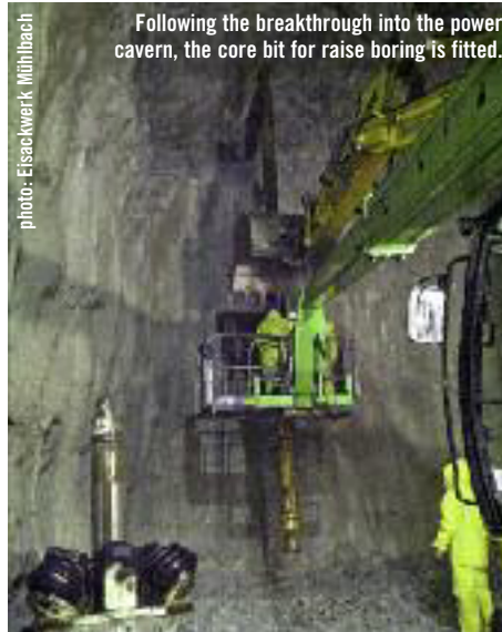
The drive rig used for the vertical bores delivers 300 kilowatts of pure excavating power.
